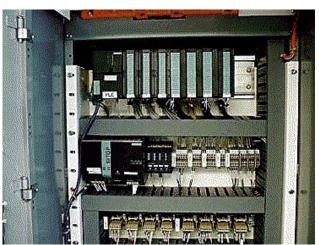
A programmable logic controller (PLC) is a specialized, self-contained computer system used in manufacturing and processing plants around the world.
